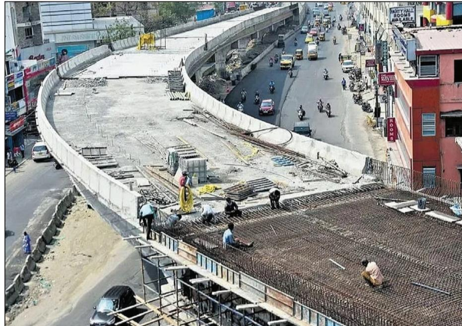
A total of 15,000 tonnes of steel structures will be used in the 3.2-km, 4-lane elevated corridor under construction on Anna Salai (between Saidapet and Teynampet junctions) at a cost of Rs. 621 crores.
